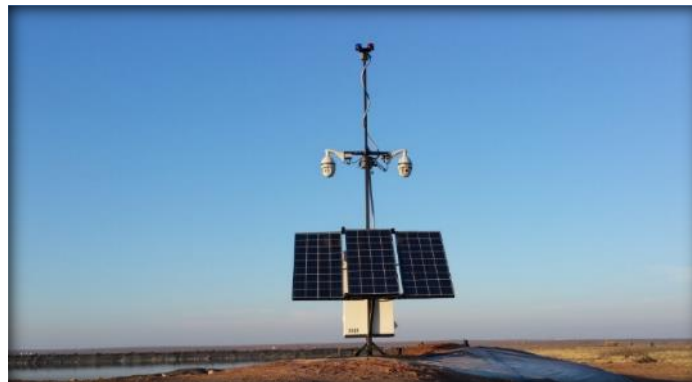
Mobile Surveillance Unit – Power Supplied by Solar Cell
